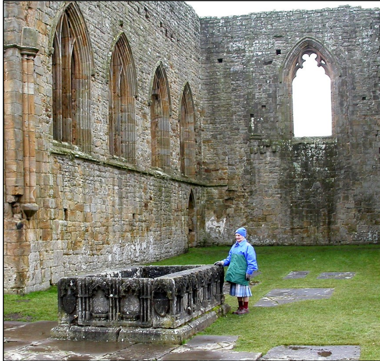
Figure 3: The monument of Sir Ralph Bowes of Streatham, (1494-1516), in Egglestone Abbey. The side stones are 0.34 x 0.7 x 3.3 metres in size. Sir Ralph fought at Flodden in 1513. The top is missing and the limestone badly weathered. [Photo: D. Goldring]
