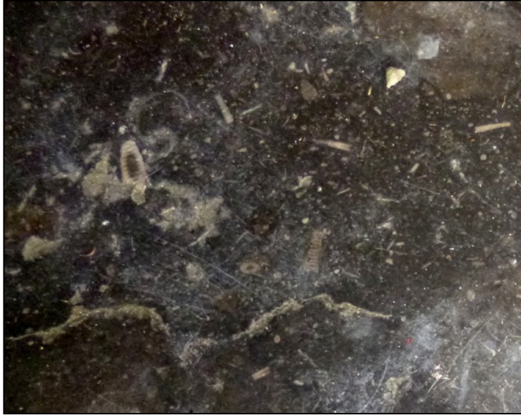
Figure 5: Egglestone Marble slab on the floor of the North Porch at St Mary's, Gainford showing disarticulated crinoid stems.
