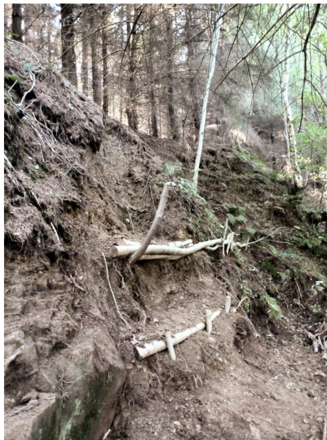
Platforms created at the new exposure to allow access to the face
